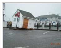
North Fork Storm Damage
